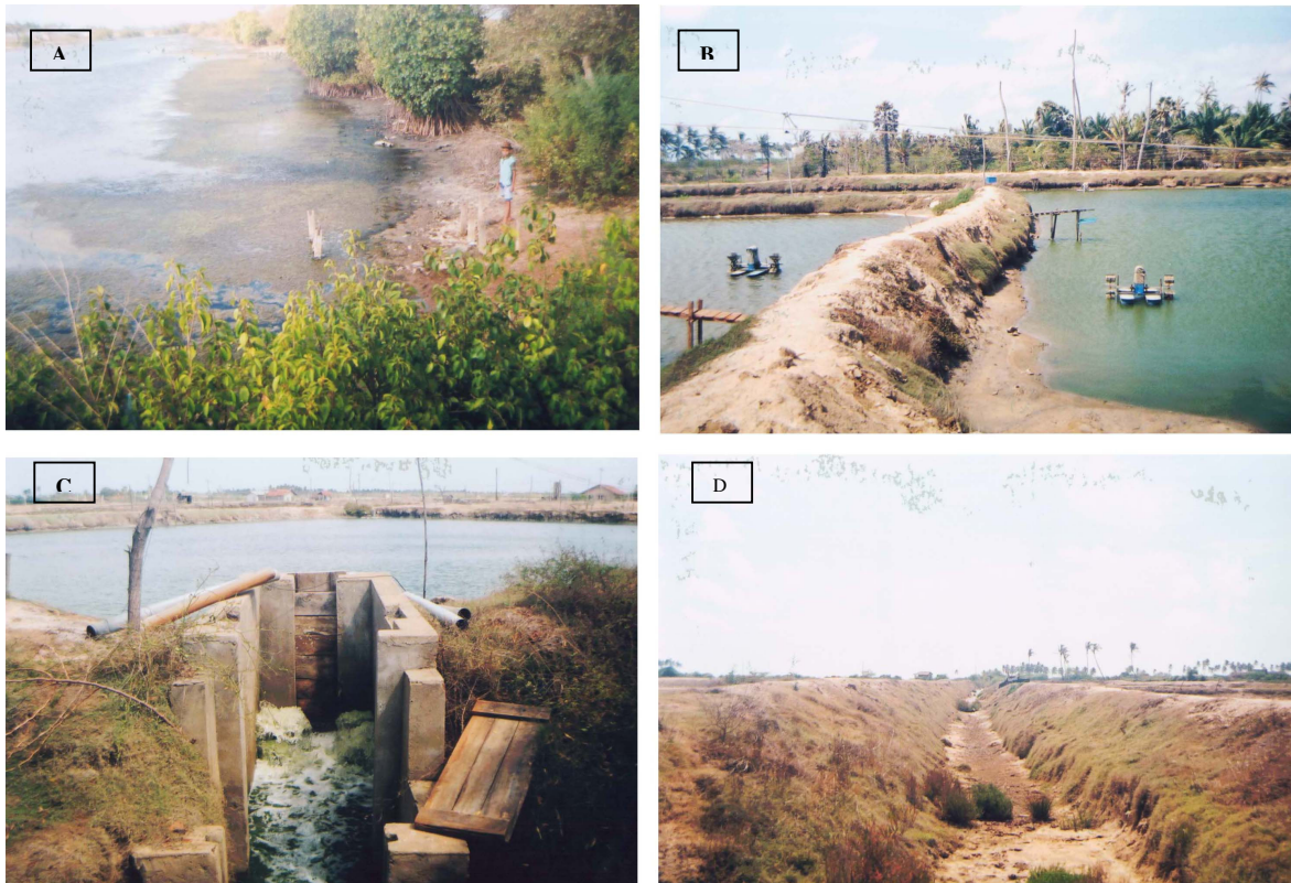
PLATE 1. Tidal flat at Muthupanitiya lagoon (A), mismanaged pond areas (B), a dam for removing of excess water as well as some effluents from the ponds (C) and manmade canal (d) in the Mundal Lake area.
