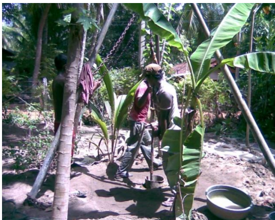
Photos 1 & 2 Hand drillings at Tube Well No. 1
